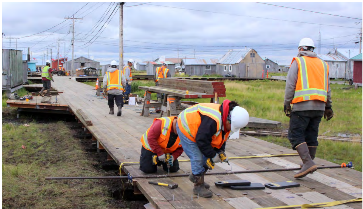
Construction workers building the boardwalk in Kongiganak in July 2016
