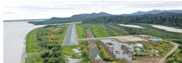
Gravel from Calista's Pilcher Mountain quarry was used this summer for emergency repairs to the Russian Mission runway that was damaged by spring flooding. Photo courtesy Brice Inc.
